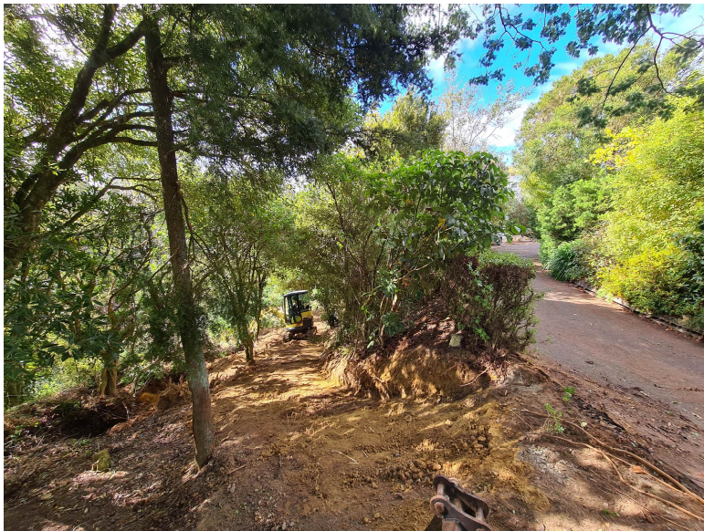
Photo 1 – Overview of the building platform on Lot 2 with accessway to right.
